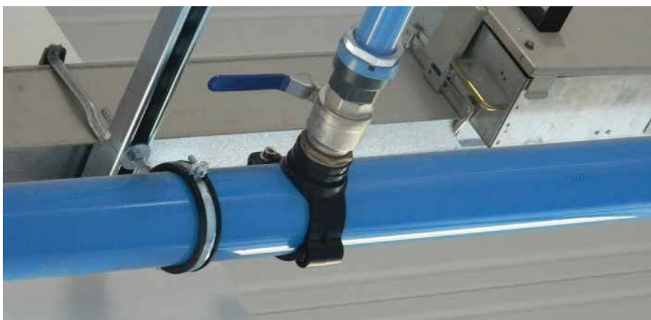
Typical Application for Saddle Branch
